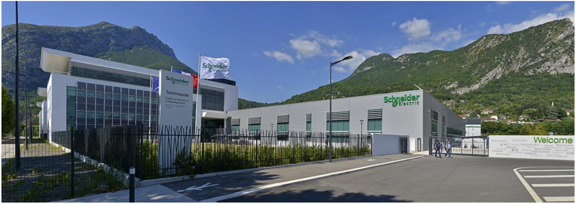
Şekil 39. Schneider Electric Technopole, Fransa (USGBC, 2020)
