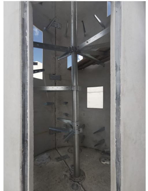
Figure 8: Construction of Volute (Photograph by Nur Gülgör, 25.07.2022)
