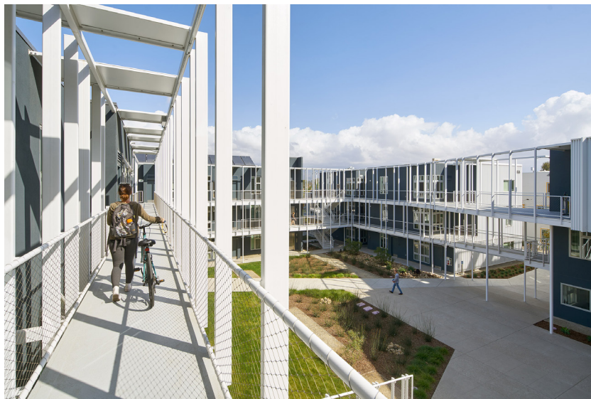
Figure 23: San Joaquin Student Housing complex/ Photography is by Bruce Damonte
