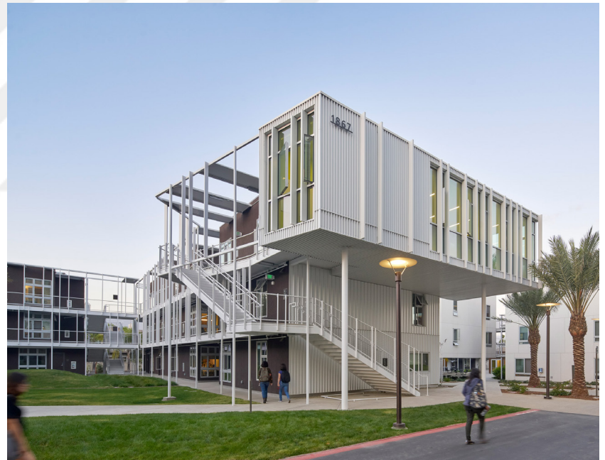
Figure 14: San Joaquin Student Housing complex/ Photography is by Bruce Damonte
