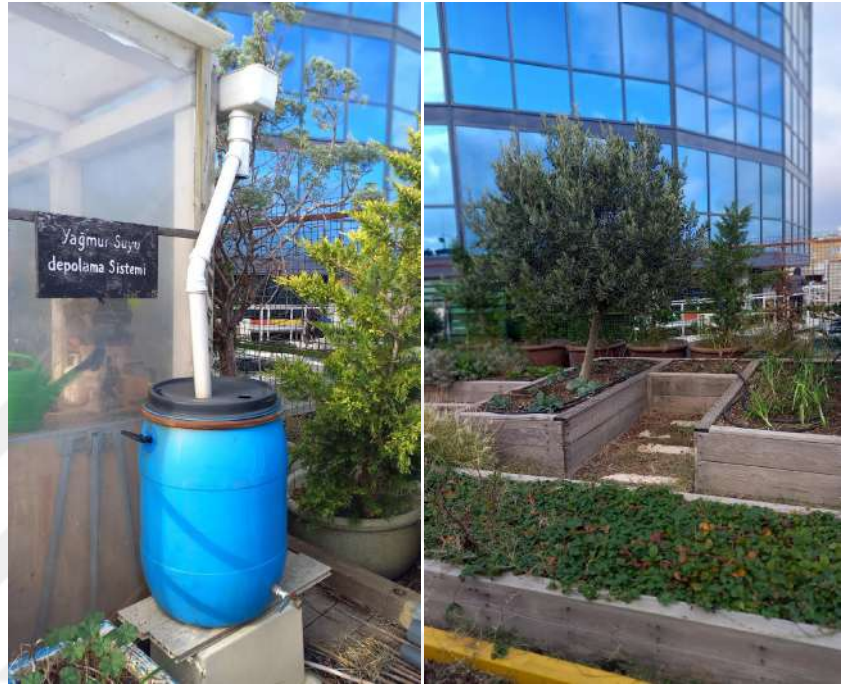
Figure 91. (Left) Rainwater storage system. (Right) A raised vegetable bed model called a keyhole. (Dilek Yürük 2022)
