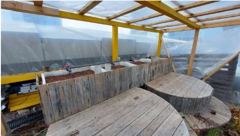
Figure 87. The structure that accommodates the aquaponic system (Dilek Yürük 2022)
