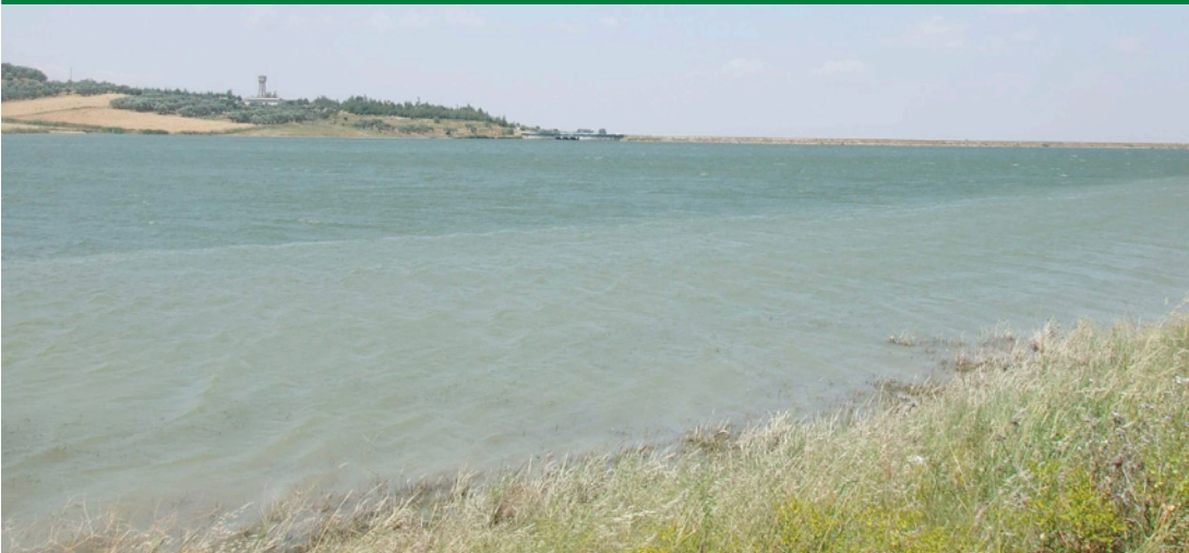
Photo 3 – Yarseli Dam (east of Antakya).
