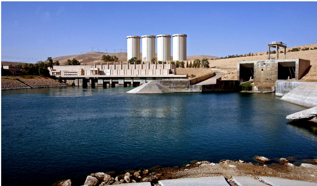
Figure 5.1. The Mosul Dam
