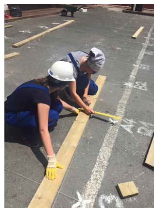
Application of the truss 1/1
