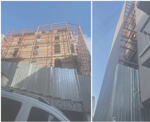
Figure 33: Building resembling intensive care unit, Lüleci Hendek St., No: 28B
