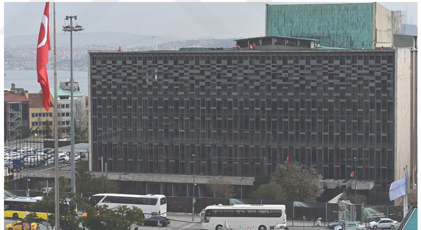
Figure 57: Idle Atatürk Cultural Center, 2013, (Source: Sözcü, "AKM yıkılıyor! Lansman pazartesi günü" [AKM is being demolished! Launch is on Monday])
