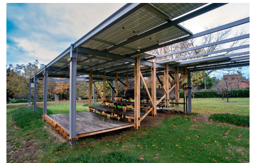
Figure 64: Yoo, Bence Güzel Pavilyon! created by reclaimed woods offers dismantling and reuse. (Source: AAP Waste Team)
