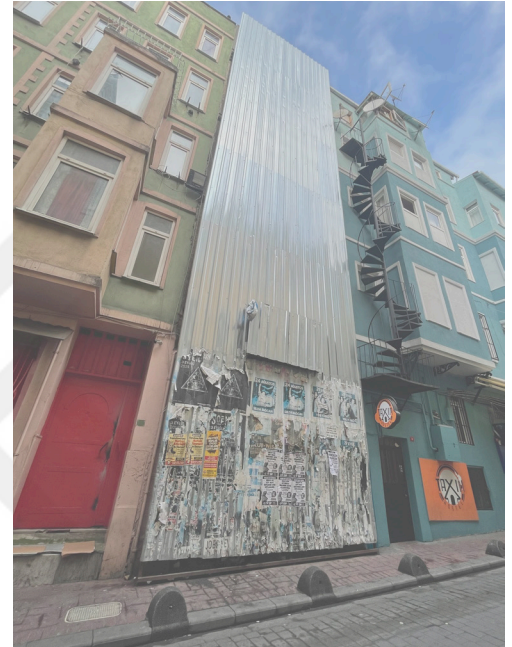
Figure 30: Building enclosed with shiny aluminum sheets, Küçük Bayram St., No: 12
