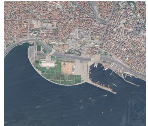
Figure 54: Yenikapı Recreation Area, built by filling with excavation waste. (Source: Google Earth, 2023).
