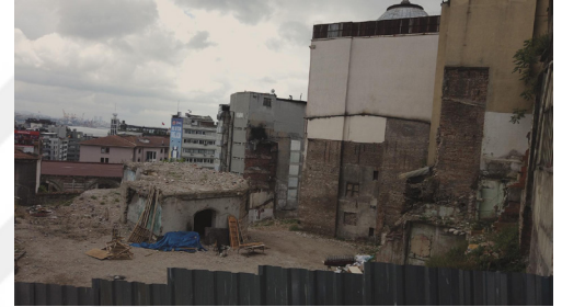
Figure 51: Mass demolitions in Zürafa Street
