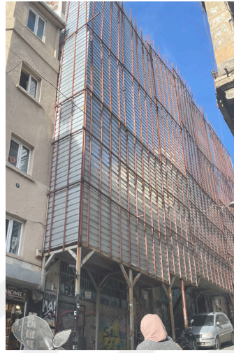
Figure 35: Building enclosed with neatly lined aluminum sheets, Yüksek Kaldırım St., No: 22
