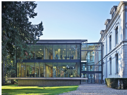
Figure 11: First building with material passport, Brummen Town Hall. (Source: Ellen MacArthur Foundation, 'A building that can be reused: Brummen Town Hall', 11 January 2022, https://www.ellenmacarthurfoundation.org/circular-examples/brummen-town-hall .)
