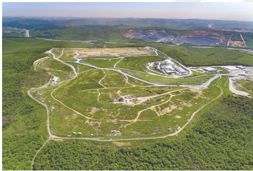
Figure 7: Odayeri Sanitary Landfill, İstanbul, (Source: İSTAÇ)
