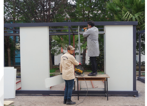
Figure 35: Students constructing a container shelter for earthquake victims, 2023. Source: Elif Özlem Çelikler- AA
