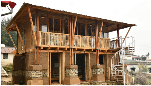
Figure 23: Compartment S4, earthquake and landslide resistant BASA Tourism Center in Khirsu, Uttarakhand, India Source: stirworld.com
