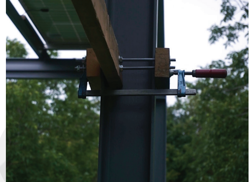
Figure 47: Compressed connector pieces stabilized with bolts, AAP MEF, 2022.
