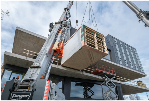
Figure 70: Construction process, placement of modular and demountable Units Source: nest-umar.net
