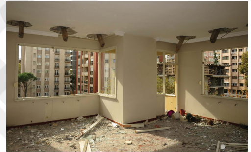
Figure 25: Selective Demolition in motion in Istanbul. Photo: Onur Ceritoğlu
