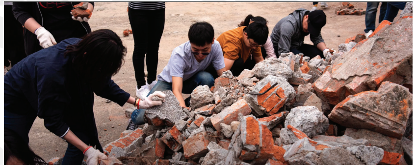
Figure 82: Participants harvesting the demolition rubble of the wall Source: C-LAB
