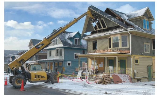
Figure 54: Deconstruction of 20th century house, 2022. Credit: Felix Heisel.
