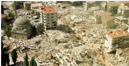
Figure 17: 1999 Marmara Earthquake Source: Politeknik
