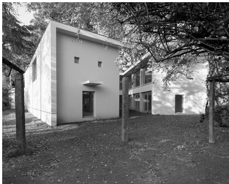
Fig. 7: Exterior view of the Carlos Ramos Pavilion
