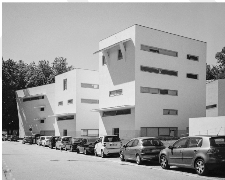
Fig. 8: Exterior view of the towers E, F and G
