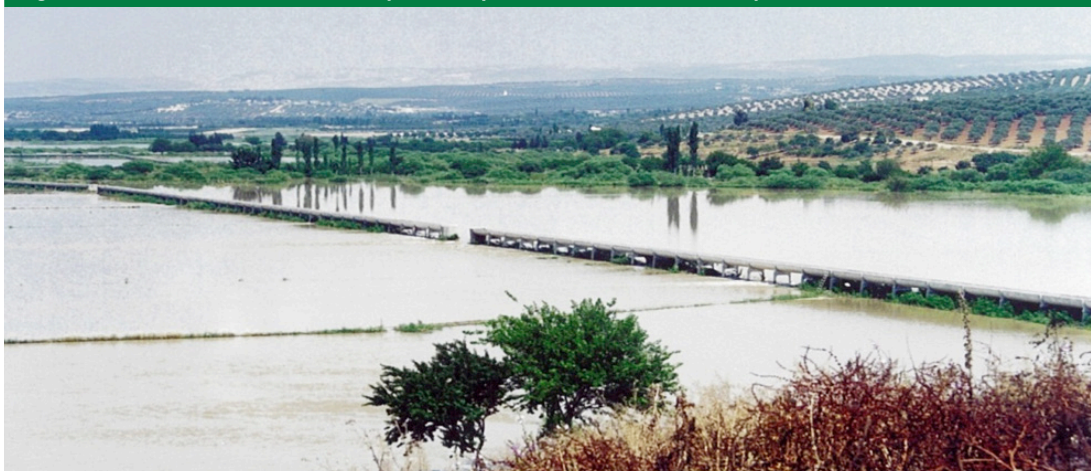
Figure 8 – Flood in June 2002 caused by the collapse of the El Zeizun Dam in Syria
