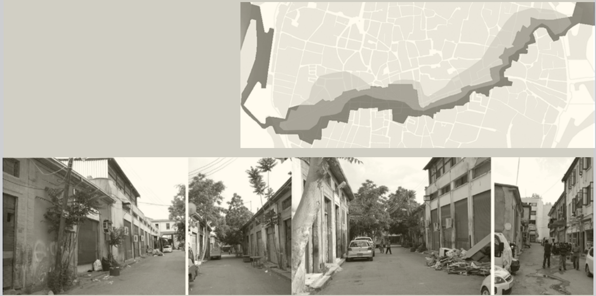
Figure 2: Decaying parts next to Buffer Zone
