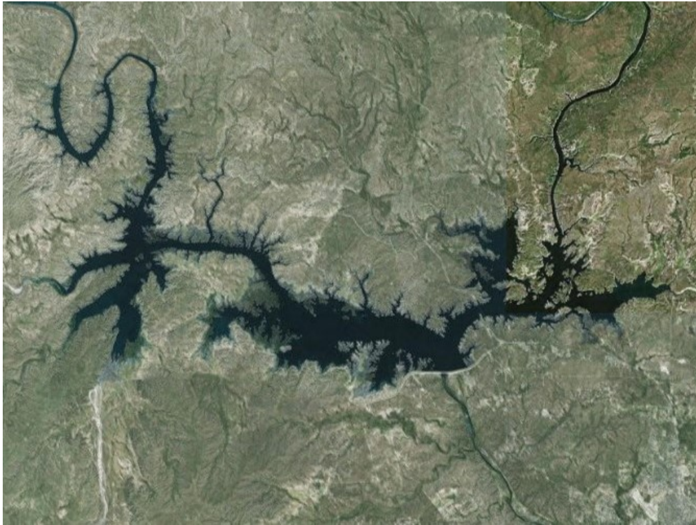
Figure 9.1. Satellite View of Amistad Dam and Reservoir
