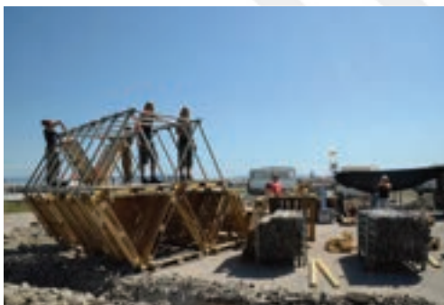
Figure 65: Construction of Hexa Structures, MyCityLab, Yes We Camp Marseille
